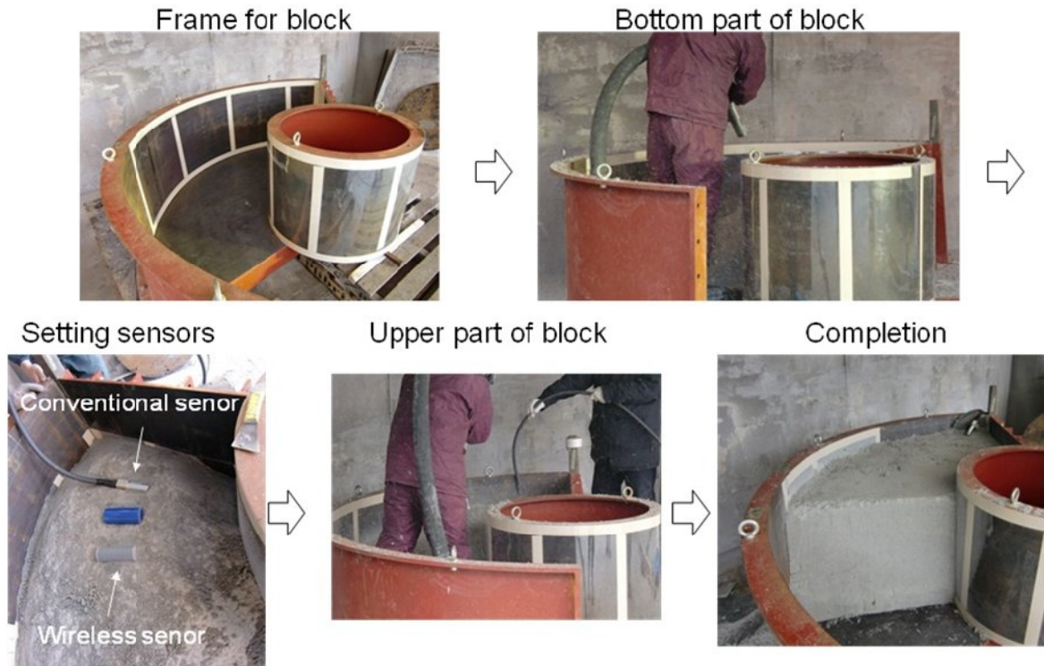
(a) Installation using the shot-clay method.
