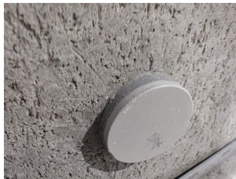
(b) Cut bentonite block around the transmitter
