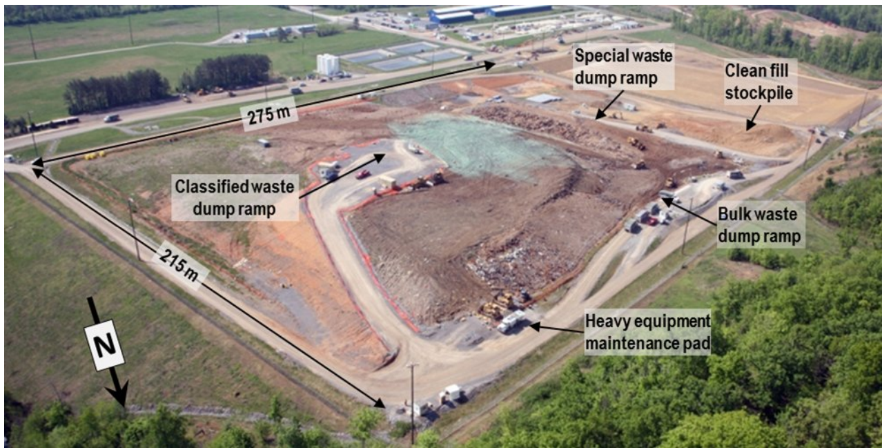
Fig 4. EMWMF facility infrastructure was developed to accommodate the standard and special waste streams being delivered.
