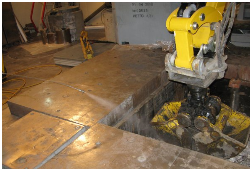
Fig.4. Removal of the equipment of loop facilities.
