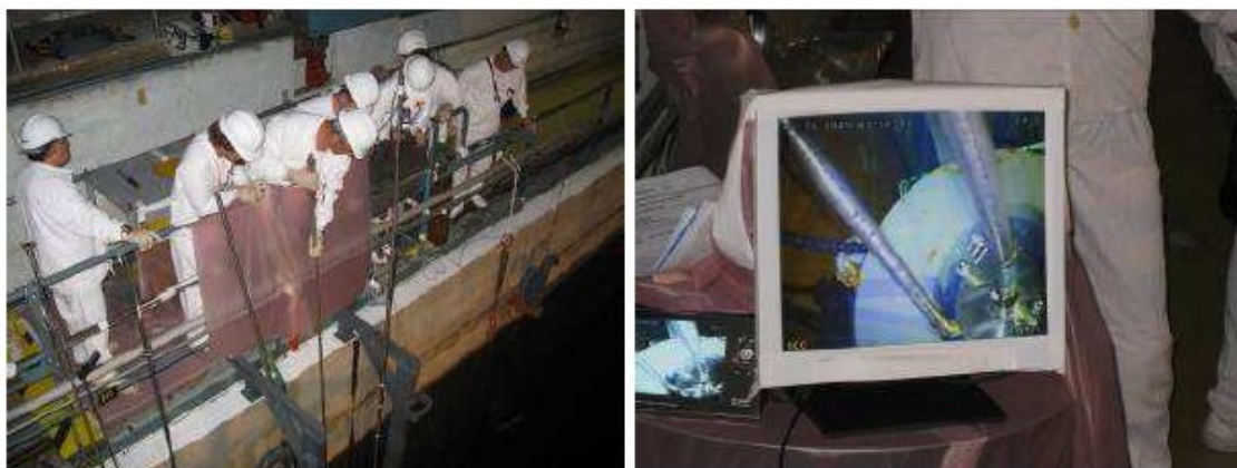
Fig 4. Closure of the primary container underwater using cameras and connection of STAUBLI poles for inerting the primary container
