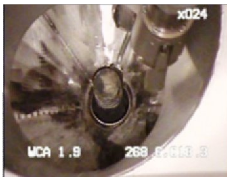
Fig 11. Inserting the slug in its transport cask and raising the package transport out of the pit
