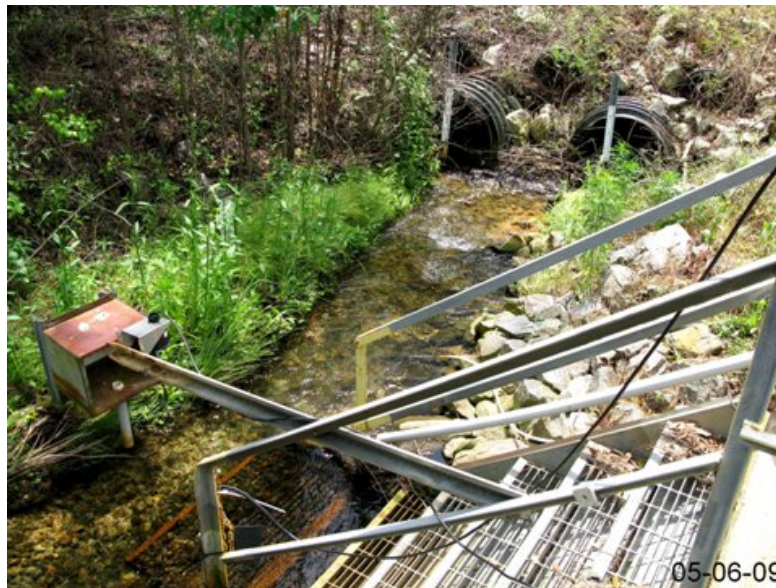
Figure 1. Typical Savannah River Site Outfall Station
