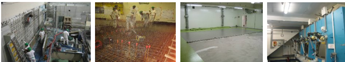
(Fig. 1) Some views of the refurbishment of the LEGS building
