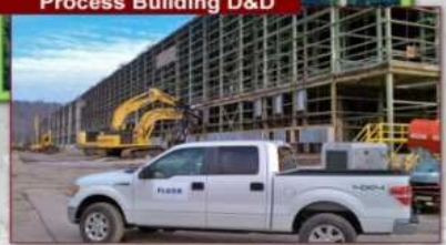
Process Building D&D
