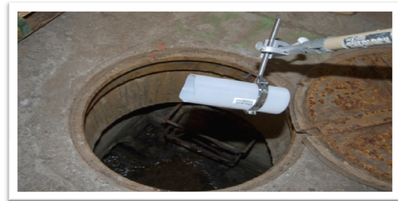
WEMA Storm Drain Effort
