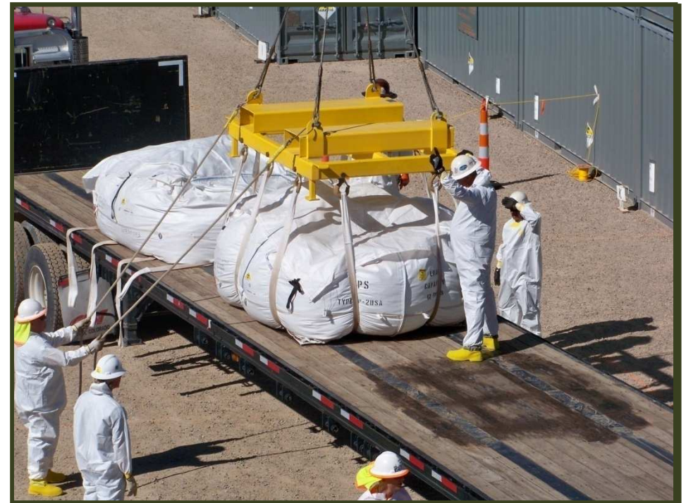
Area 5 Offloading Super sack Shipments with Enhanced Contamination Controls in Place
