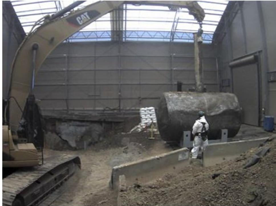
Tank W-1A removed January 6, 2012
