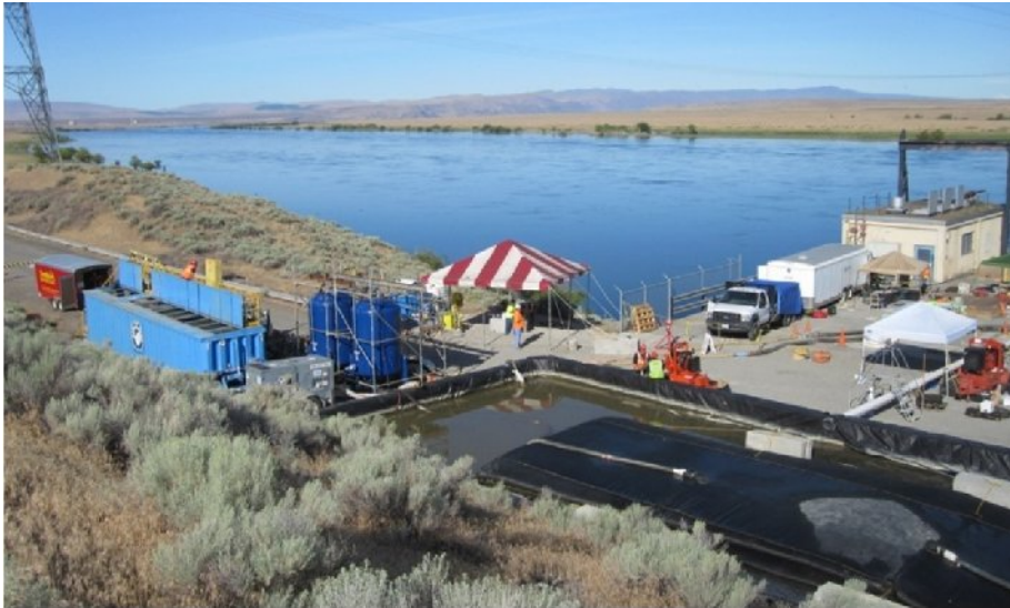
Sediment removal at N Reactor river intake structure
