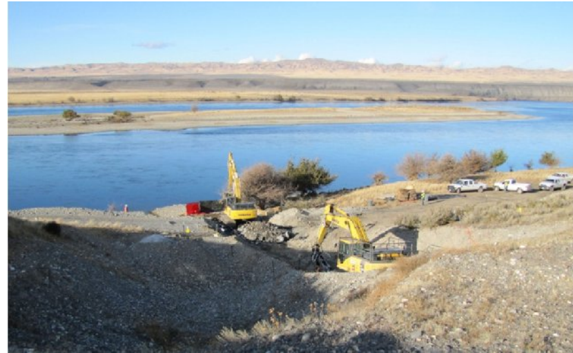
Waste site cleanup along the Columbia River
