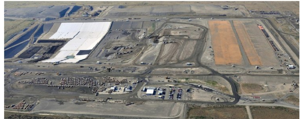
Environmental Restoration Disposal Facility expansion was completed ahead of schedule
