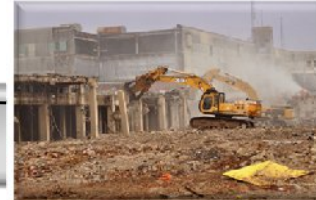
2008: Building K-25 West Wing demo begins
