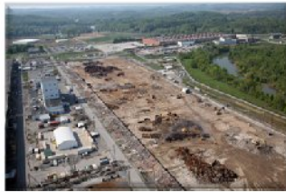
2010: Building K-25 West Wing demolished
