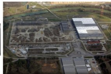
2011: Building K-33 at ETPP demolished
