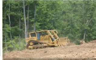
2007: Expansion of onsite disposal facility complete
