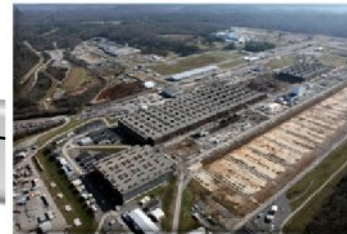
2011: Began Building K-25 East Wing demolition
