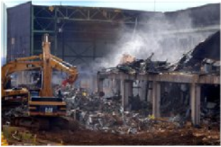
2006: Building K-29 at ETPP demolished
