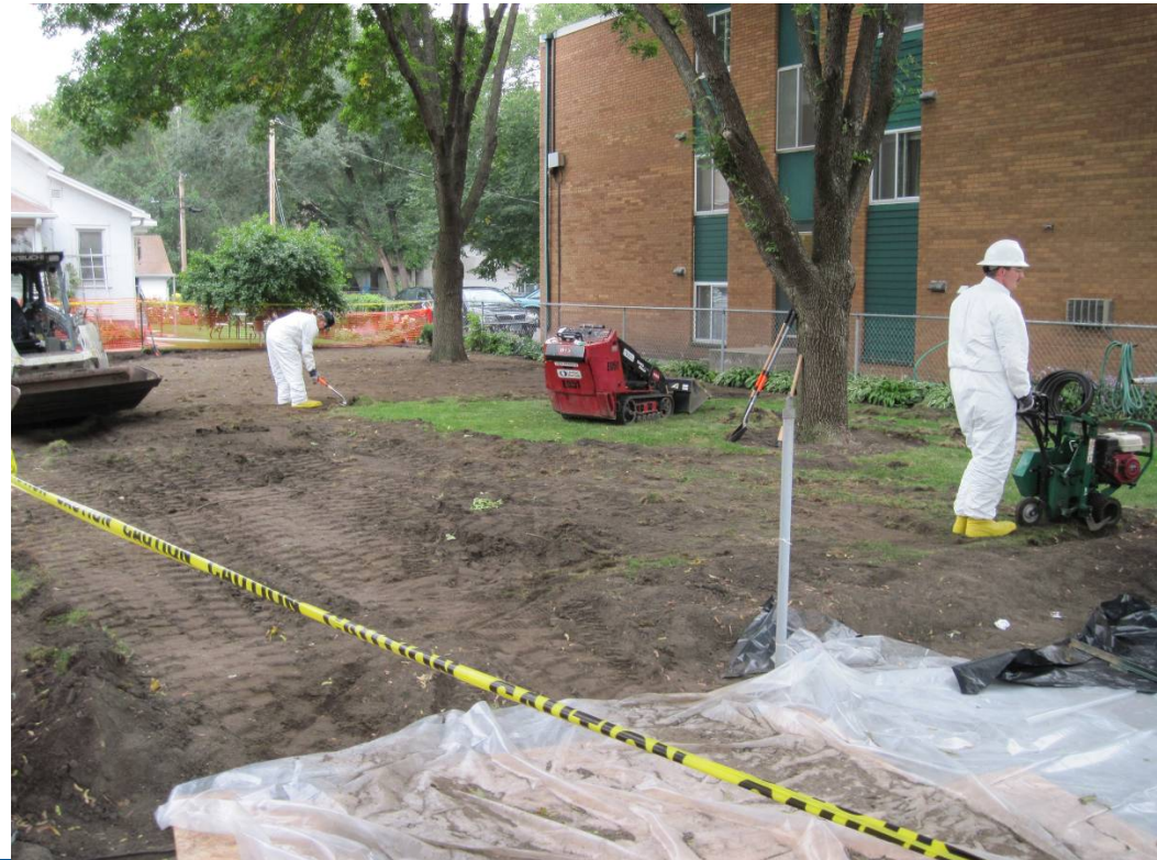
EPA residential area remediation
