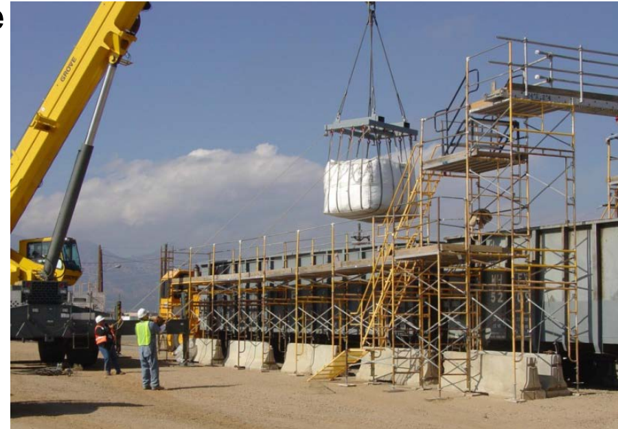
Loading waste into railcars for transport
