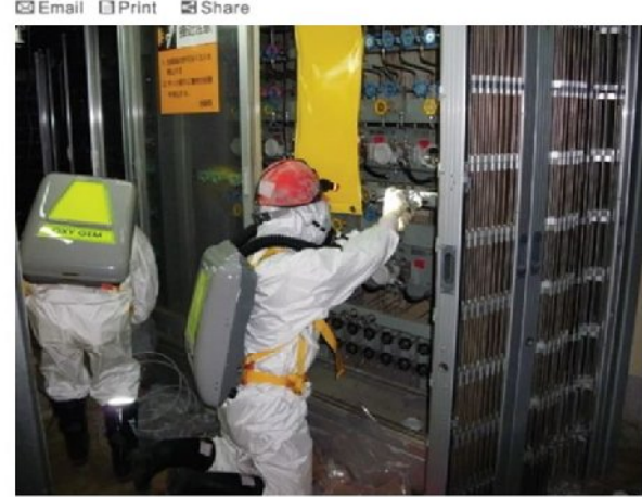
DOUBLE CHECKED: Workers at Fukushima Dai-ichi reactor 1 check a water level indicator. Injected water has cooled the cores, but it has also created contamination at the site.
