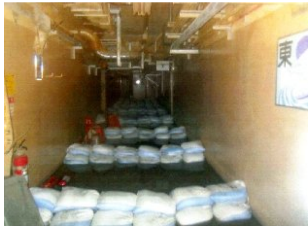
High Temp Incinerator Building
