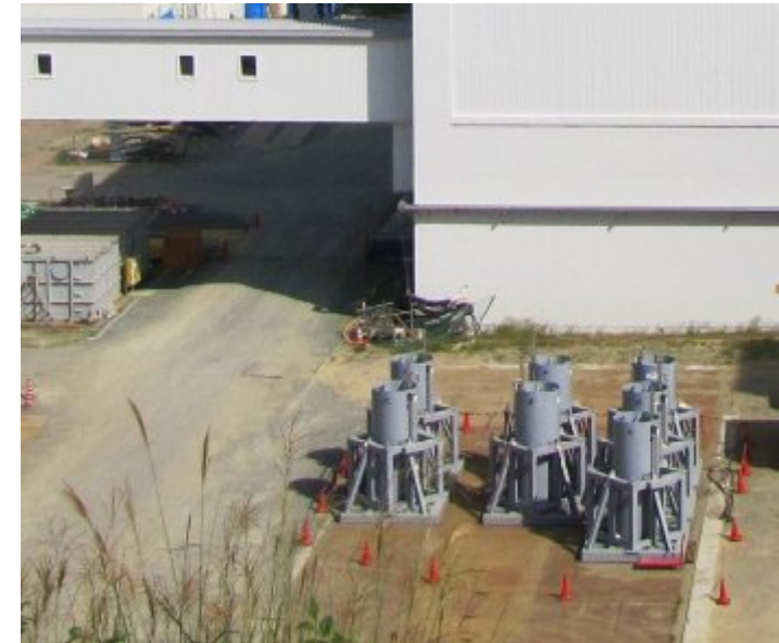
Shielded Ion eXchange Module (SIXM) Storage
