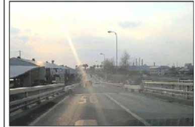
Miyagi prefectural road, Route 240 East Japan Railway, Miyagi Prefectural Government
