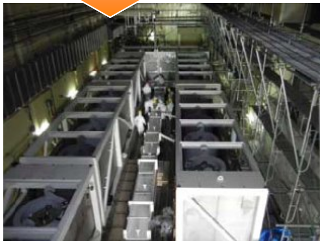
Cesium Adsorption Tower
