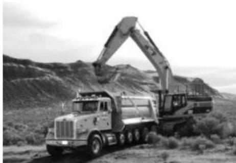
Right – A super dump truck is loaded with soil for disposal. The trucks provided increased capacity with reduced worker handling.
