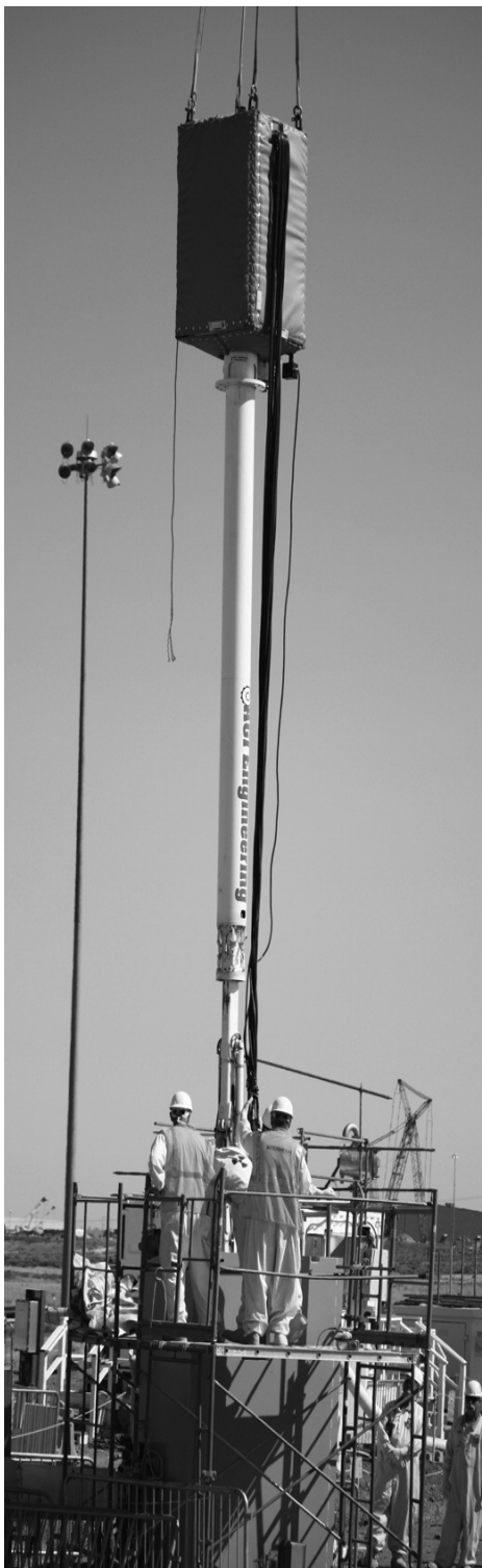
Hanford workers install a modified sluicer into Tank C-112, one of two tanks currently undergoing waste retrieval. The Enhanced Reach Sluicing System shown here fires a high-pressure stream of liquid via a telescoping arm that extends further down into the tank than more traditional sluicing methods.
