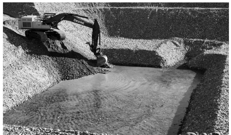
Backhoe removed contaminated soil at Hanford
