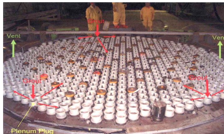
Figure 8. Top of the P-Reactor Plenum.
