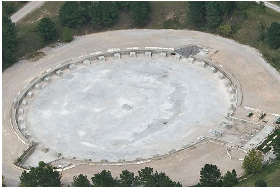
Site Cleaned and Restored
