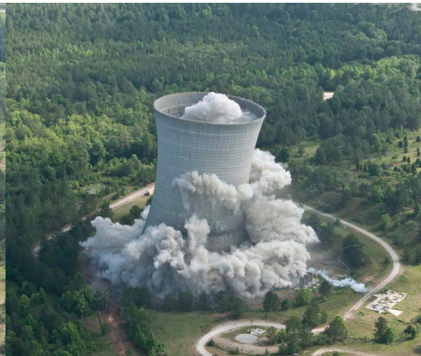
Foundation Support Failure
