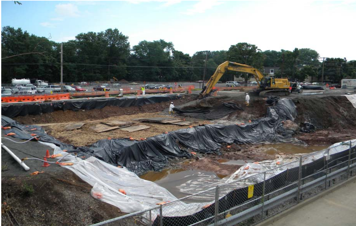
Figure 2. Ongoing remediation at NRC-licensed Burial Pit 2 in July 2010.
