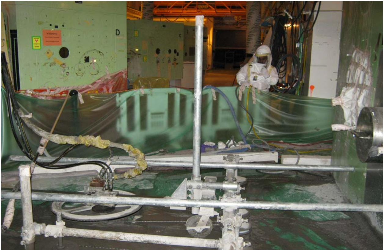
Figure 2. Wiresaw Cutting of Upper SERF
