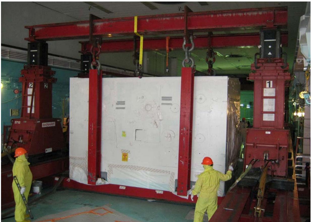
Figure 3. Removal of Hot Cell from Building
