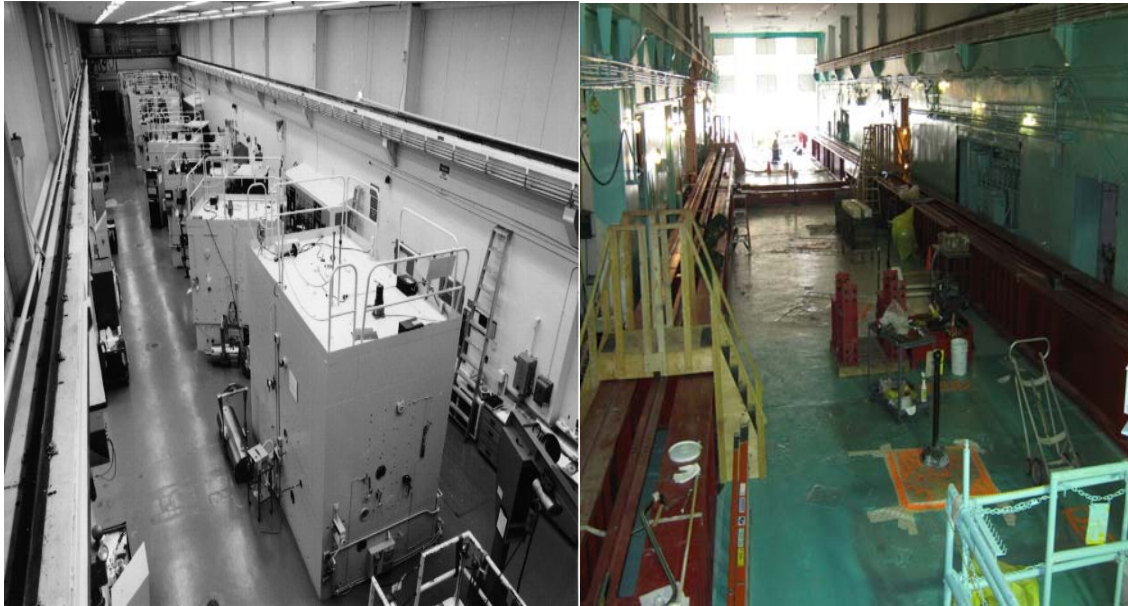
Figure 1. First Floor Layout Before/After Hot Cell Removal
