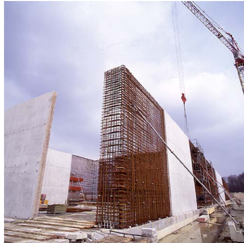
Figure 9: disposal vaults under construction at Centre de l'Aube disposal facility (LIL-SL)
