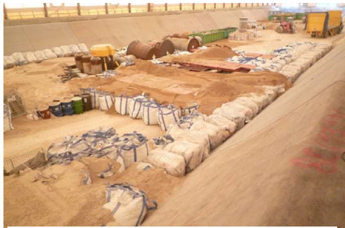
Figure 6: disposal cell with sand backfilling
