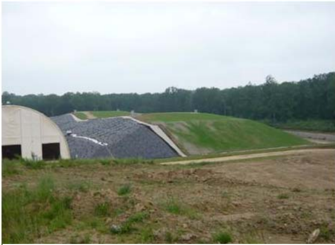
Figure 3: implementation of the capping system
