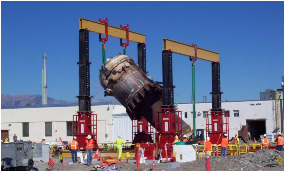
Figure 1: Lift of the ETR Reactor Vessel using a Gantry Crane.
