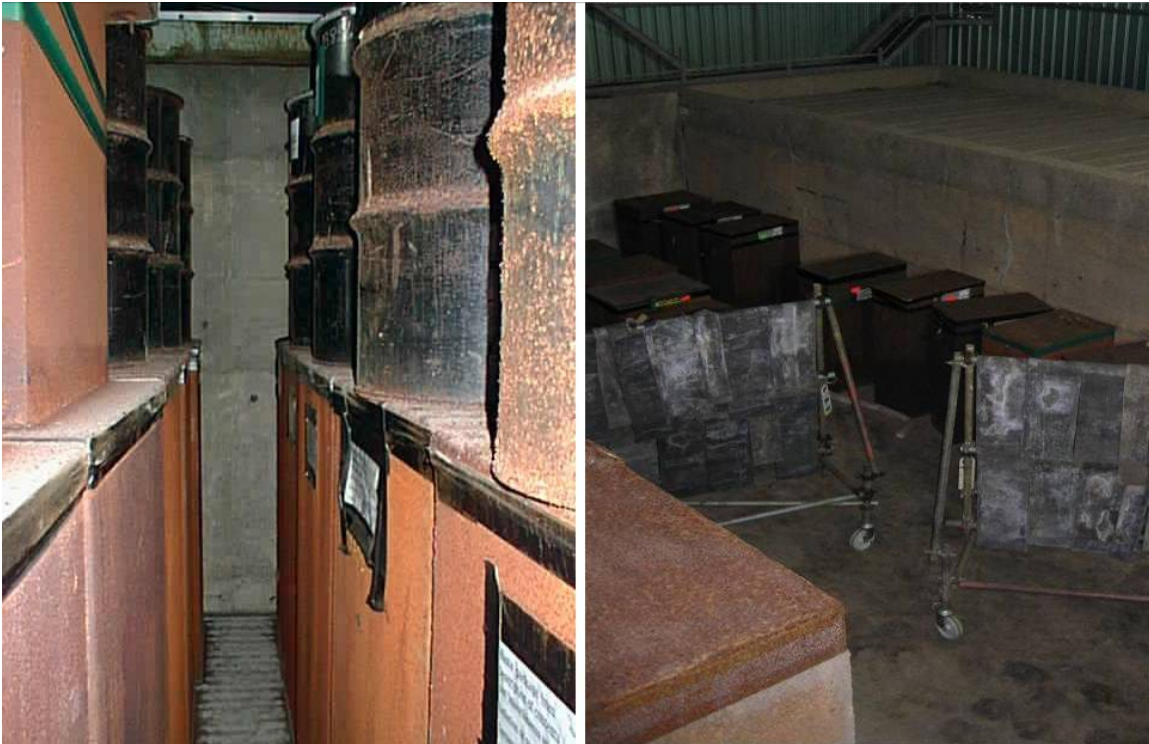
Fig. 2. Accumulation of ILW and PCM waste items in the Inter-Cell areas.
