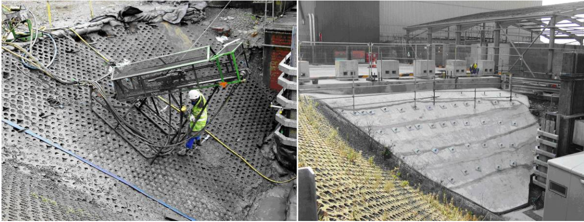
Fig. 3. Soil Nailing operations (left) and a section of completed batter (right)
