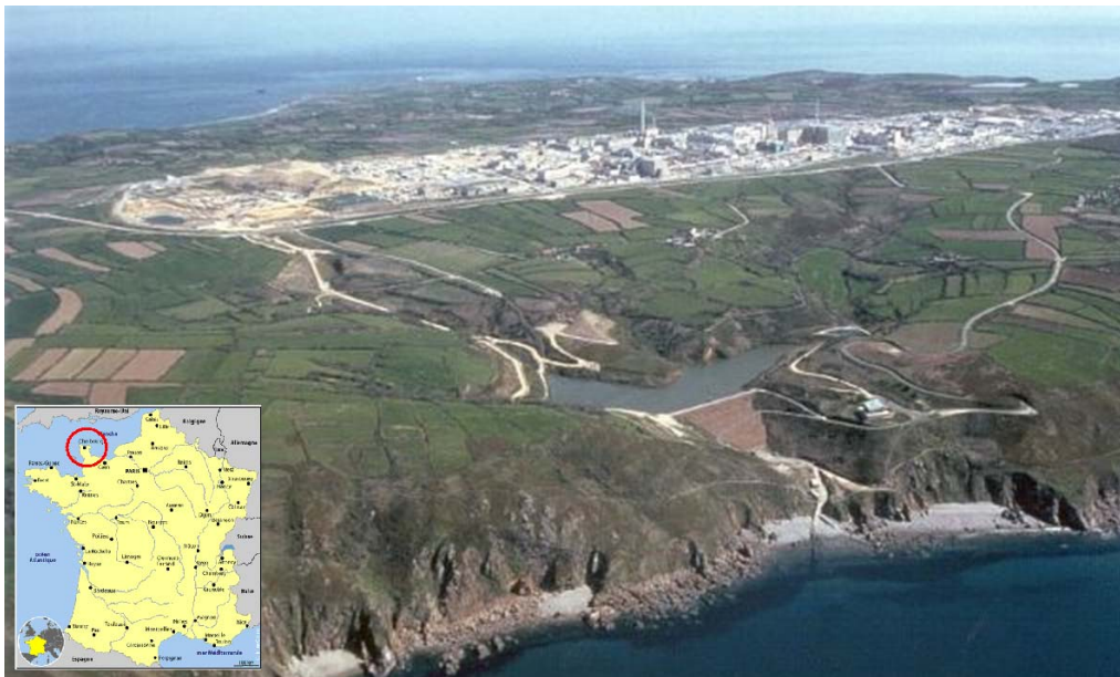
Figure 1: Areva La Hague plant, including interim storage facilities on right side
