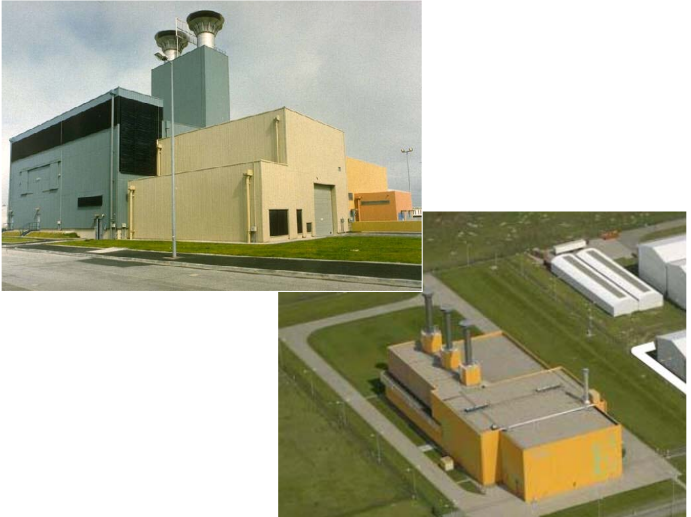
Figure 4: View of the E/EV/SE installation and of COVRA Habog facility
