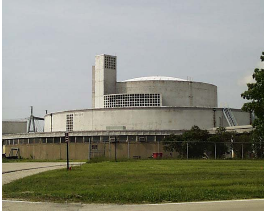
Figure 1: Building 330 at Argonne National Laboratory
