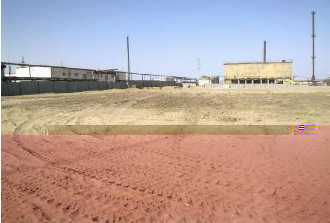
Fig. 8. Balkanabat Iodine plant charcoal adsorption shop site appearance after remediation.
