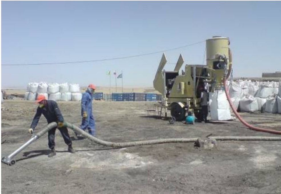
Fig. 6. Waste collection with the industrial vacuum cleaner.
