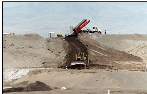
Fig. 4. A truck dumps waste into ERDF. In 2008, an average of 150 truckloads of waste was disposed per day. In 2010, more than 650 truckloads were disposed on some days.
