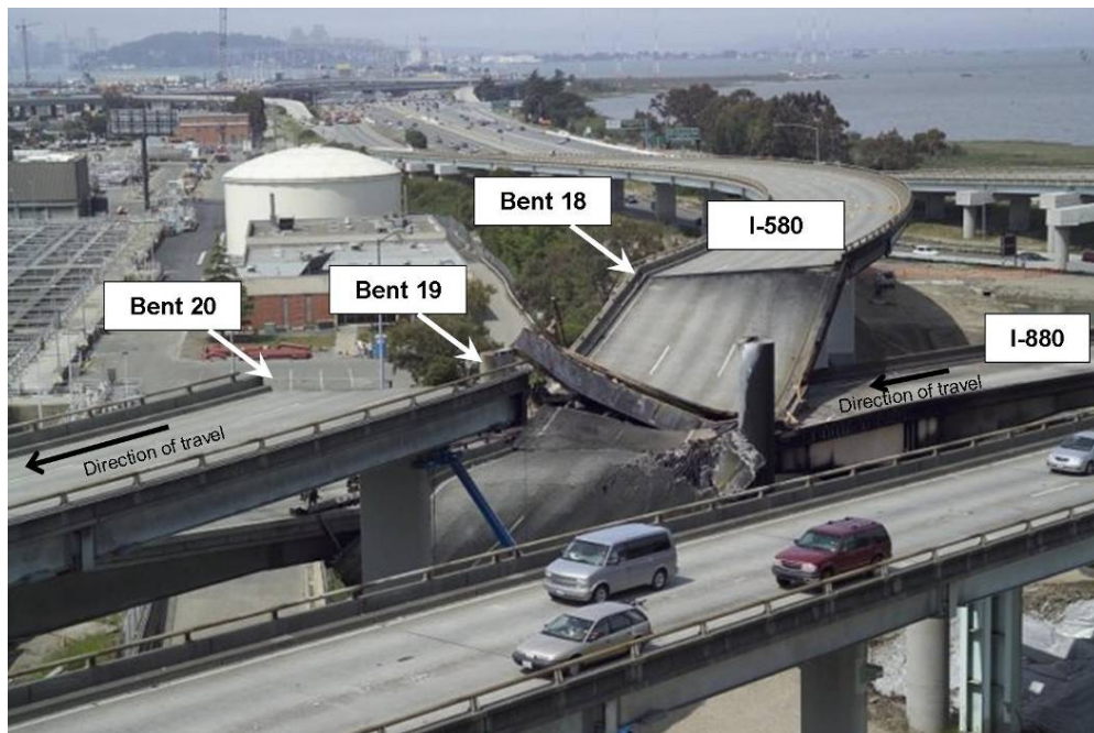
Fig. 2. Post-fire aerial view of the collapsed section of I-580 looking west. Picture from Caltrans http://www.dot.ca.gov/dist4/photography/images/070429 .
