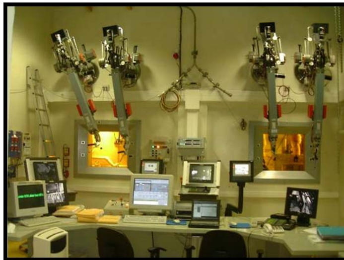
Figure 1 – Control Station with Waste Sorting Manipulators In Background
