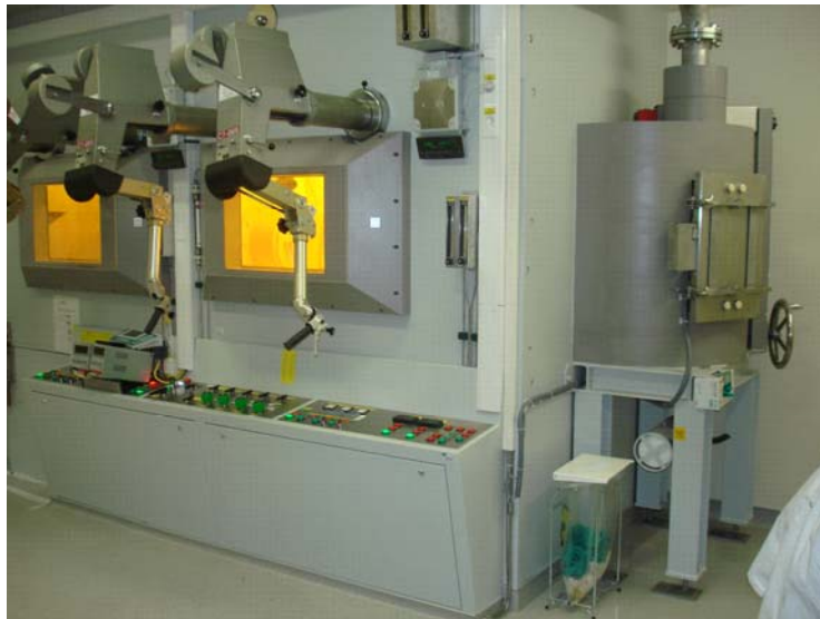
C7 Cell after renovation
