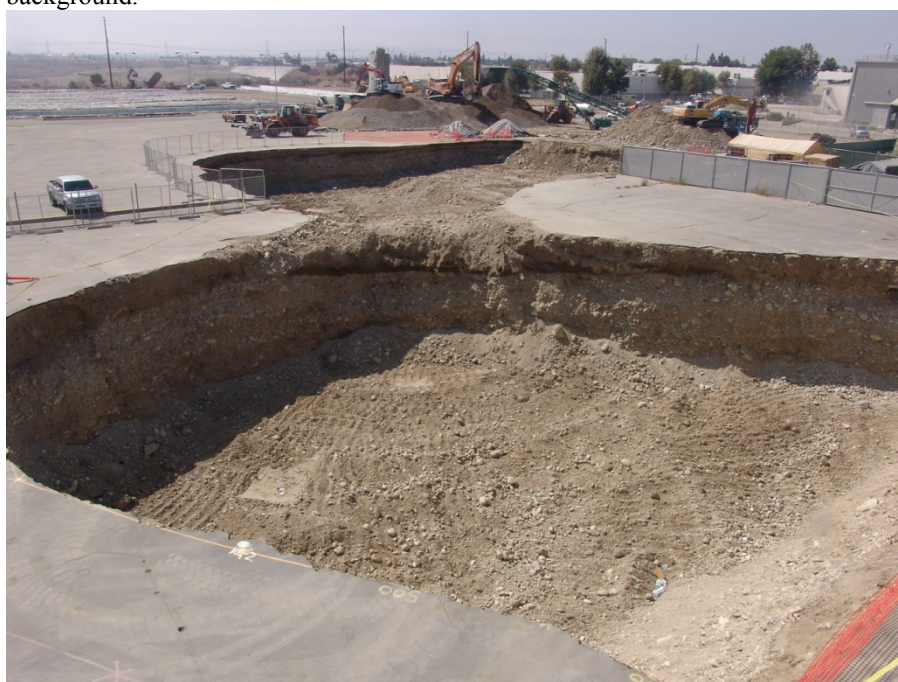
Figure 3. Completed Excavation with Soil Processing and Biotreatment Cells in Background.
