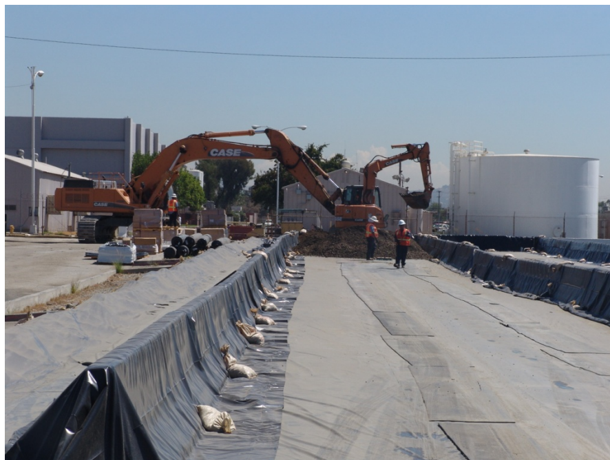
Figure 4. Loading of a Biotreatment Cell
