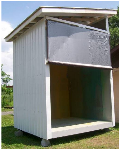
Fig. 2. Building module at ICM facility.
