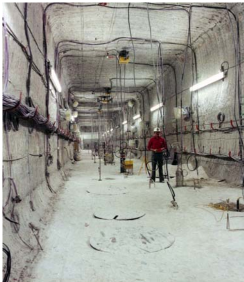
Figure 10. Vertical placement of heaters simulating HLW at WIPP[16].
