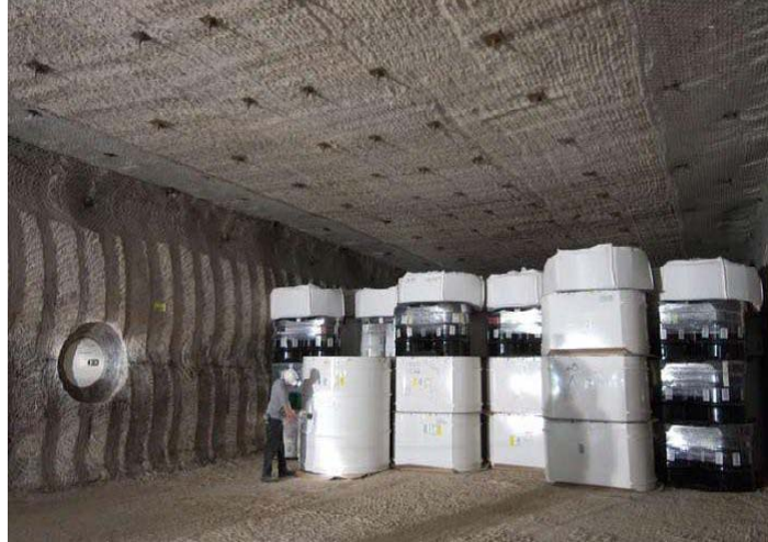
Figure 9. Disposal configuration for transuranic waste at the WIPP.
