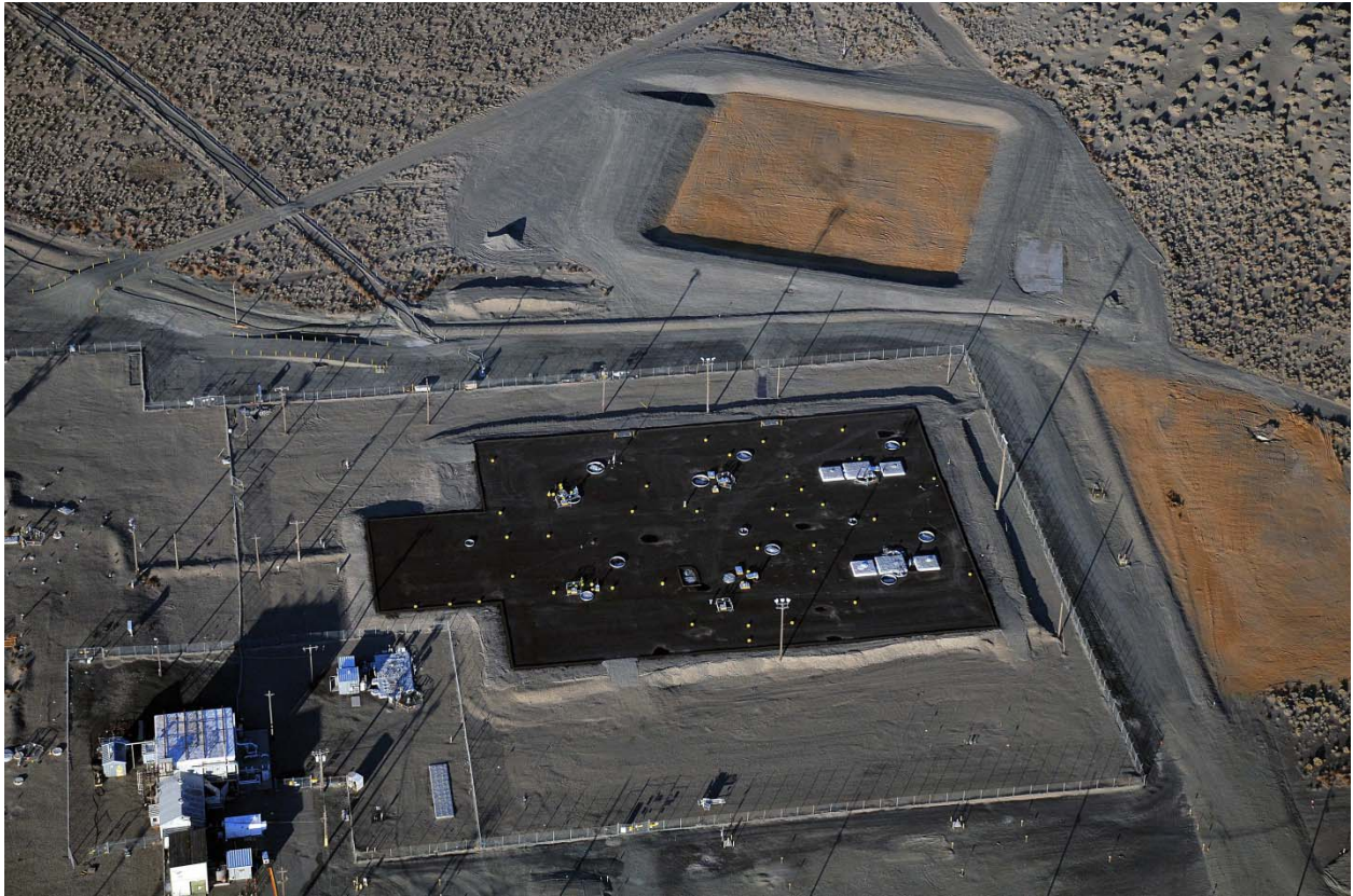
Fig. 8. Photograph of final barrier.
