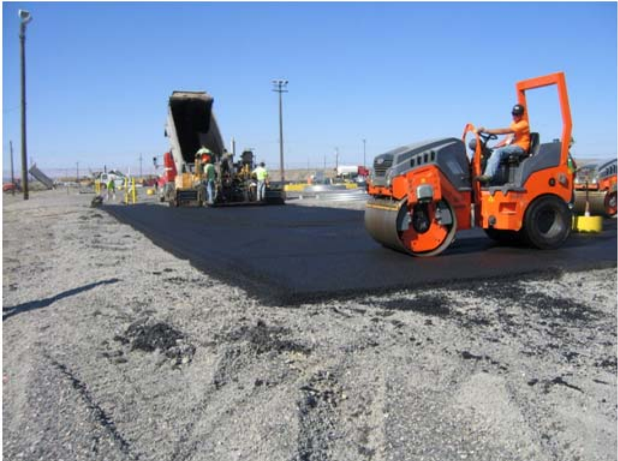
Fig. 7. Photograph of asphaltting.
