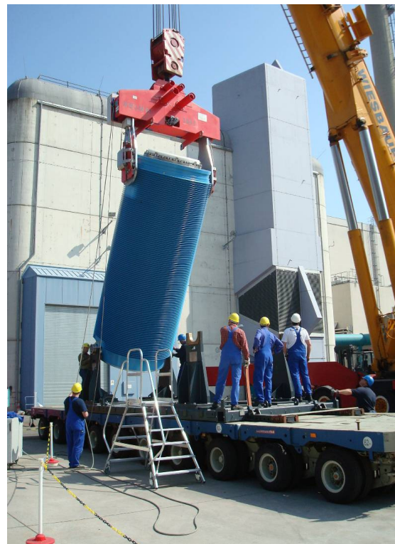
Fig. 4. Handling of a CASTOR cask outside of the VEK
