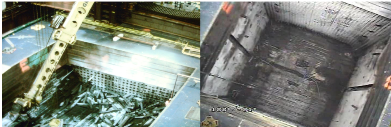
Fig. 4. Bucket/thumb tool extended down into the cavity by excavator arm – mining
