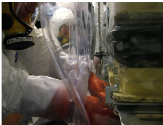
Figure 1 Transfer Tunnel Separation
