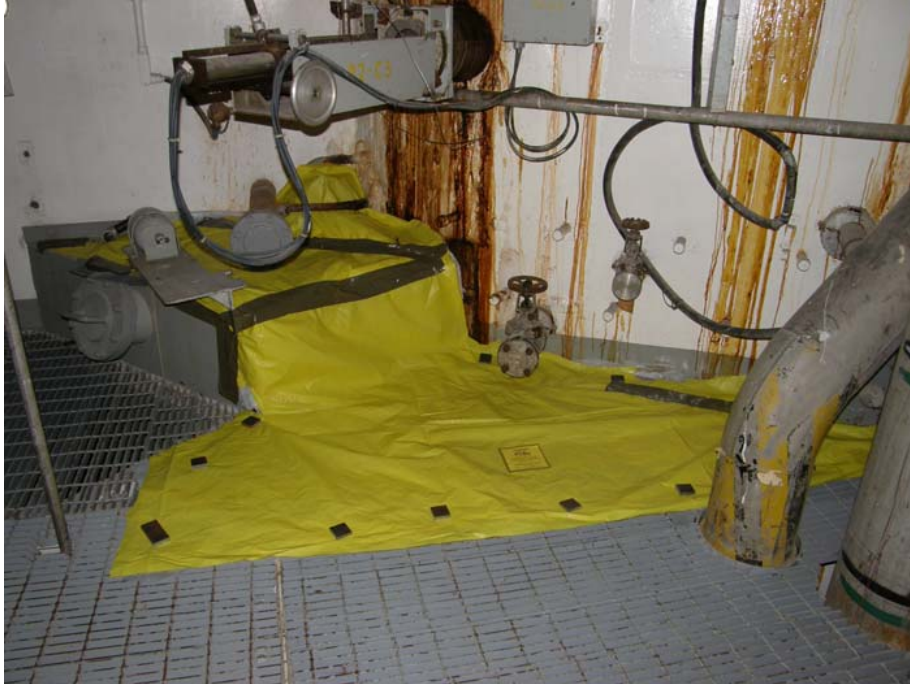
Figure 3. This photograph was taken in building 105-L at the -20 elevation where the horizontal surfaces have been cleaned by scraping, covered and labeled.
