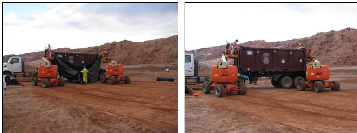
Fig. 2. Disposable plastic liner installation in a container.
