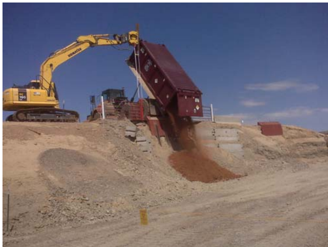
Fig. 4. Excavator with vibrator attachment releasing holdup.
