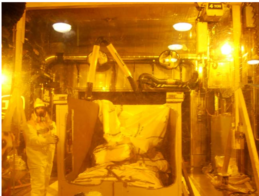
Fig. 4. CSRF cutting room. Note flexible exhaust Plymovent ® arms in the top center of the photo.
