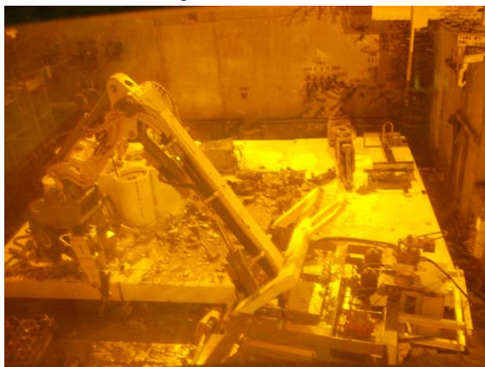
Fig. 2. Floor plates within the VF to make space usable. BROKK ® 330 in the foreground, and cutting table in lower left corner.
