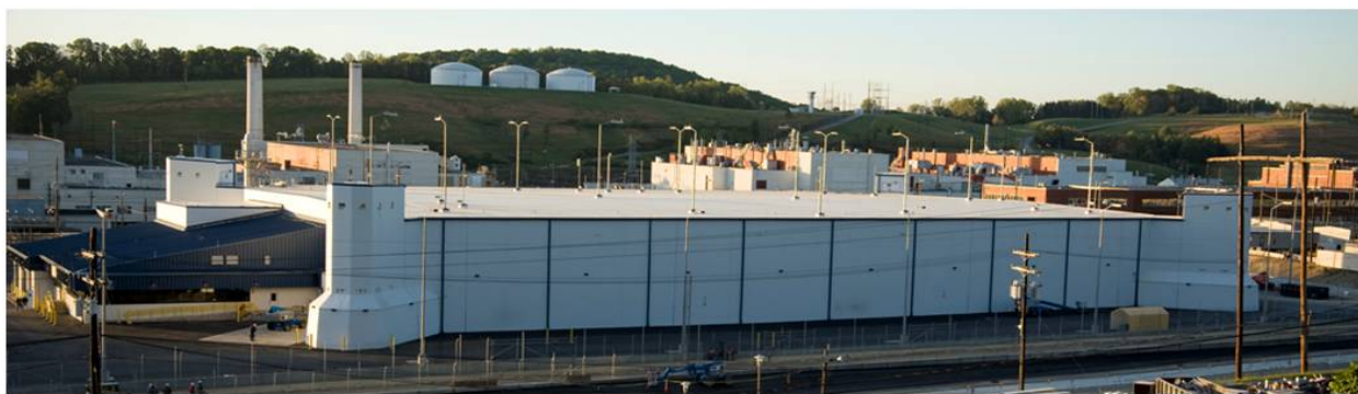
Fig. 2. The Highly Enriched Uranium Materials Facility securely stores the nation's stockpile of highly enriched uranium that is not in a nuclear weapon.
