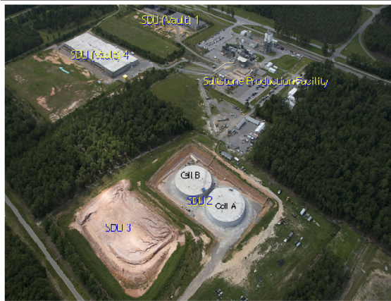
Figure 1.C: Saltstone Production Facility
