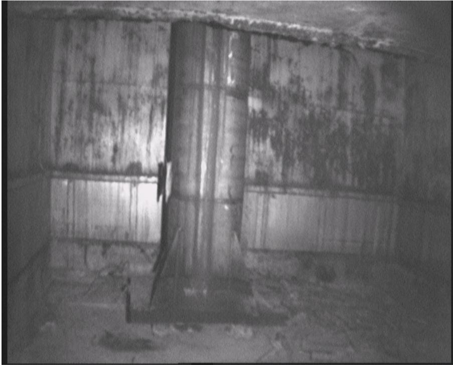
Fig.1. Photograph from video survey showing waste container and debris field (to the right) in the waste vault underneath the BN-350 hot cell.
