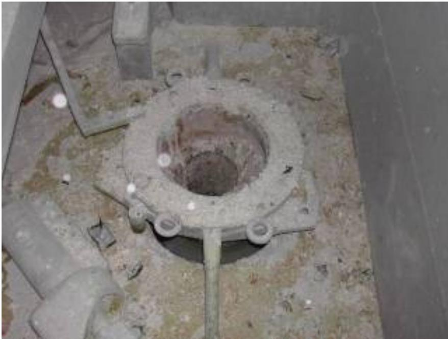
Fig. 5. Photograph of access point into spent fuel drum, taken during man entry into the fuel transfer box, showing oxidised deposits of sodium
