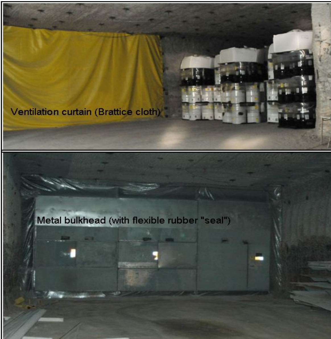
Fig. 2 Photos of a typical ventilation barrier called a brattice curtain (top) separating each disposal room, and of a typical metal bulkhead (bottom) “sealing” the inlet and outlet drifts of each disposal panel from ventilation air in the rest of the mine.
