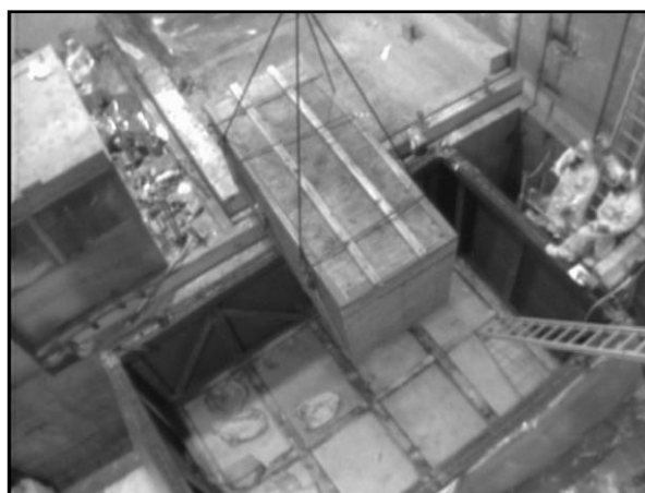
Removing plywood boxes
