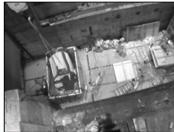
Ductwork moved to SLB for disposal
