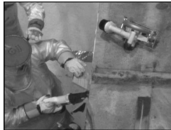
Cutting access window for contamination check
