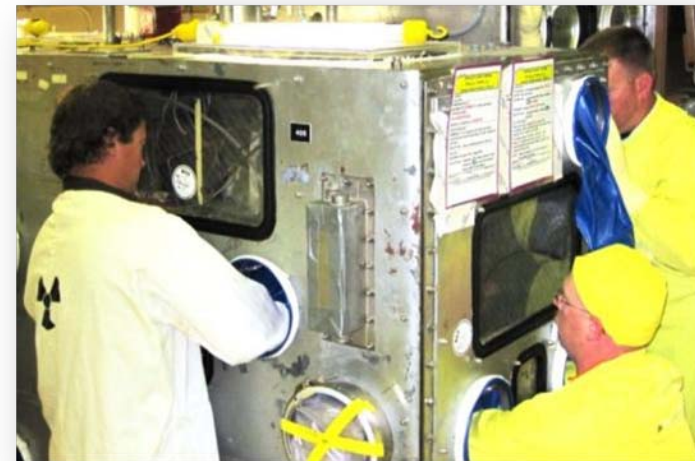
Workers Mock-up Process Equipment Removal in a PFP Glove Box
