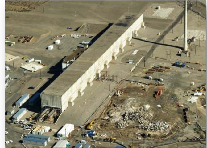
U-Canyon Ancillary Facilities after Demolition
