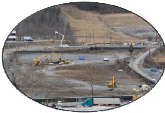
Old Salvage Yard 94% complete
